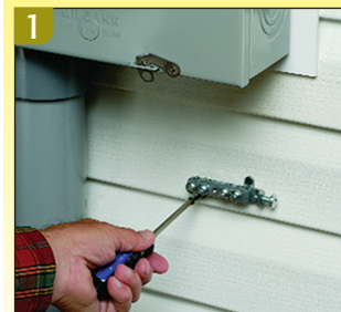
1 Attach bridge to substrate. (Mounting screws not provided.)
