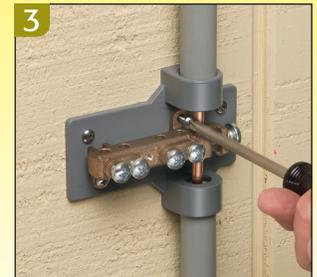
3 Insert grounding electrode conductor into the lay in lug. Tighten screw.
