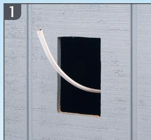
1 Cut a 3-1/4" x 5-1/2" hole in substrate. Pull wiring.
