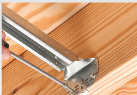
Bracket mounts securely to joists.
