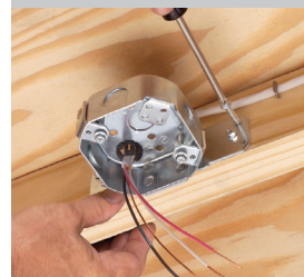
FBS415S/FBS420S Mount on SIDE of Joist
