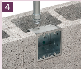
Install the EMT in the top of the box.
