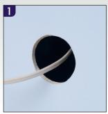
Cut hole with a 3-1/4" standard hole saw and pull wire. Push box through drywall. Built-in "teeth" create a path for device screws.
