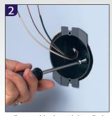
Pull NM cable through installed connector. Tighten bracket screws inside box to seat bracket securely against drywall.
