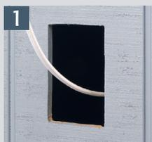
1 Cut a 3-1/4" x 5-1/2" hole in substrate. Pull wiring.
