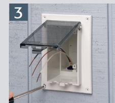
3 Attach IN BOX with stainless steel screws (provided).
