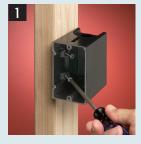
Attach ONE-BOX to wood or steel stud with captive installation screws. If the box is too far forward or back, simply back the screws out and reposition.
