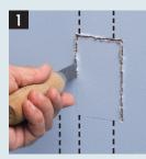
For old work position ONE-BOX adjacent to stud. Use box as the template to cut hole.
