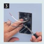
Mount ONE-BOX directly to stud with shipped in place screws.
