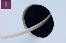
1) Cut hole with a 3-1/4" standard hole saw and pull wire. Push box through drywall. Built in "teeth" create a path for device screws.
