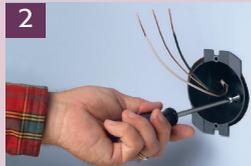
2) Pull NM cable through installed connector. Tighten bracket screws inside box to seat bracket securely against drywall. Create a path for device screws.
