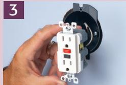
3) Install device (GFCI shown) and maxi size cover plate (not provided).
