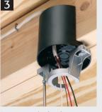
Remove captive bracket installation screws. Use them to mount fan/fixture bracket. (Installation of drywall not shown.)
