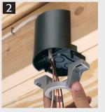
Position mounting bracket over locator posts to assure proper position. Pull wires through KO.
