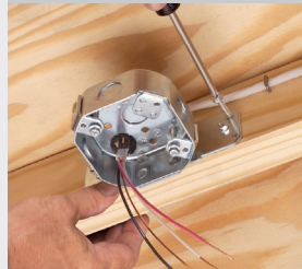
FBS415S/FBS420S Mount on SIDE of Joist
