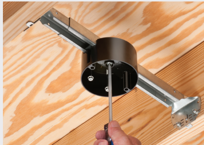
Loosen center screw to position box on bracket.
