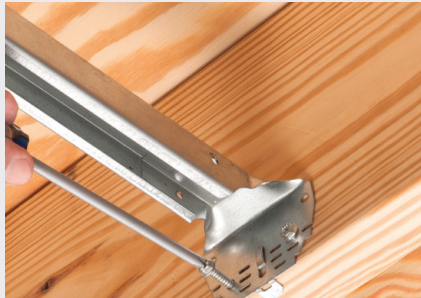
Bracket mounts securely to joists.
