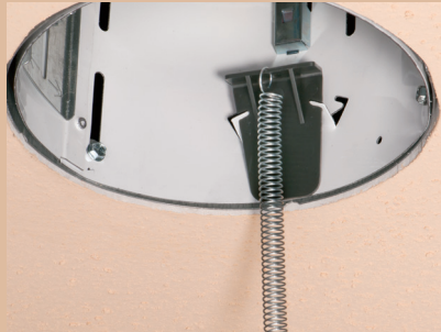
Installation Method A, Slip plastic anchor brackets into the tabs in the 'can'.
