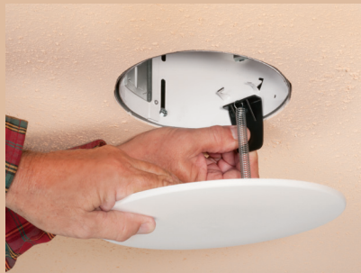
Attach the anchor brackets or extension springs to the inside of the 'can'. Tension on the springs pull the cover plate snug against the ceiling. Paint cover as desired to match ceiling.
