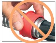
2 If you are using an end stop bushing, determine which one to use by sizing it to the cable bundle (not the metal jacket). Incorrect size shown above. The metal jacket should never go through the end stop.
