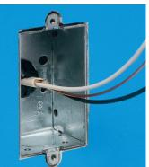
A box this shallow does not allow for the installation of larger devices.
