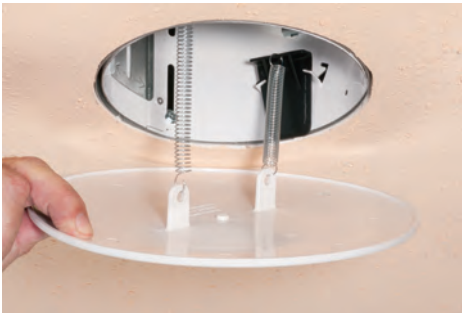
Attach the anchor brackets or extension springs to the inside of the 'can'. Tension on the springs pulls the cover plate snug against the ceiling. Paint cover as desired to match ceiling.
