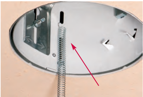
Installation Method B No tabs inside the can or too close to fixture. Attach the springs directly to the 'can'.
