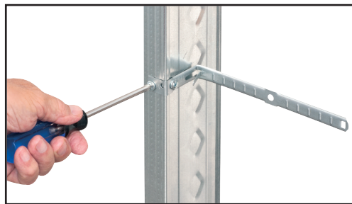
1 Nail or screw CUS6 support to metal or wood stud (metal shown).
