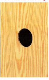
1 Cut hole in substrate with a 4-1/2" hole saw.
