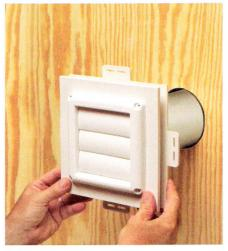
2 Insert vent tube into opening.
