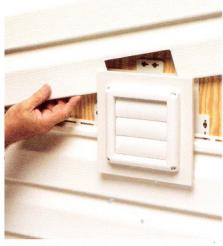
4 Install siding. Overhang on vent flange hides cut ends of siding.
