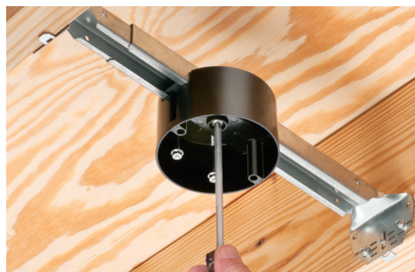
Loosen center screw to position box on bracket.
