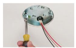
Center box in hole. Tighten sled to hex. Pull cable through NM cable connector and remount box to the bracket. Attach fan/fixture bracket to box using the supplied screws.
