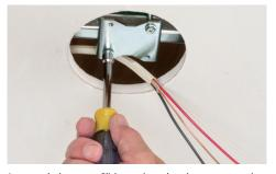
Loosen sled screws. Slide to along bracket to access the hex bar. \*\*There is no need to remove the sled.
