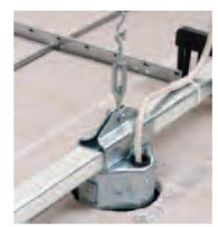
Cable pulled thr ough installed NM cable connector.
