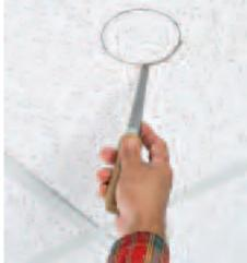
1 Cut a 4-1/16" diameter hole in the center of a 24" ceiling tile.
