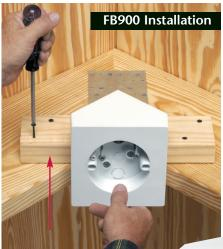
Cut a 2x4 approx. 14" long to span rafters. Install FB900 in center, then attach the 2x4 to the rafters, keeping bottom of box level, and short sides of box touching angled rafters.
