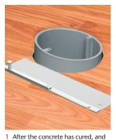
the flooring is installed, use a saw to cut the box...
