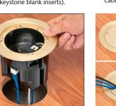
6 Place FLBR5420 Floor Box into hole. Orient the box to suit installation. Tighten four wing screws to secure box to the floor.
