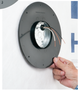
Place flashing backing over box.
