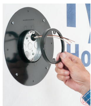
Using two supplied #8 screws, attach appropriate ring to installed box. FR410F comes with two rings; one for a pan box, the other for an octagonal box.
