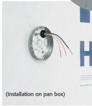
Mount box to sheathing after the installation of weather barrier.
