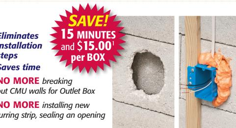
Arlington's new Furred Wall Box™ saves time - and makes challenging outlet box installation easy!
