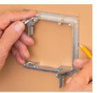
One or two-gang bracket is the template for cut out. Level. With the new design it's easier than ever! Make a pencil dot in the notches in each corner. Draw a line
