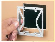
4 Cut opening. Insert bracket into opening.
