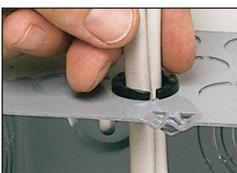
**2** Insert one or two cables in a single opening, fast! Push the NM cable(s) into the connector to the desired length.
