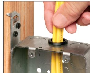
**2** Insert one or two cables into individual openings.
