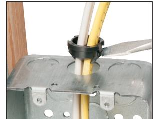
**3** To remove from KO. Slip screwdriver under connector and twist.
