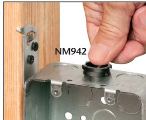
**1** from **OUTSIDE** new work box Push NM942 into KO with light finger pressure.
