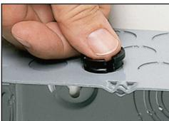
**1** from **OUTSIDE** box push the NM cable connector into KO with light finger pressure.
