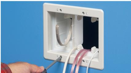
3 Tighten mounting wing screws to pull the box securely against the wall.
