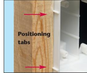
2 Positioning tabs are set for 1/2" and 5/8" drywall. Install NM cable connector. Pull wires.
