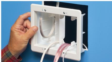
2 Cut drywall. Attach trim plate to box (screws supplied.) Pull wire/cables. Install assembly in hole.
