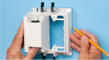
1 Use enclosure (*without trim plate*) as a template for opening. Cut 5-1/4" x 6" hole.
