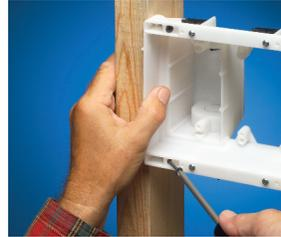
1 Attach box to stud using supplied screws. Use tabs on box for proper positioning of box depth.
