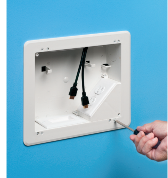
Tighten mounting wing screws to pull box securely against the wall.
