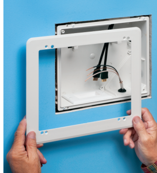
Attach trim plate with screws provided.
