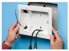
4 Install trim plate. Pull cable through connector. To install box in hole tighten wing screws (see 3).
