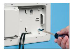
7 OPTION Attach box to block for added stability.
