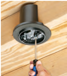
1 Screw to joist
