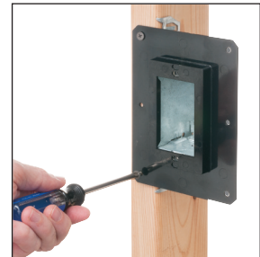
...or the flashed-over holes to hold the vapor box cover in place during drywall installation.
