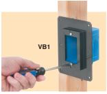
Use the supplied #6-32 screws through the device screw holes...
