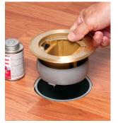
2 Secure the leveling ring assembly to the installed FLBC4500 can with PVC cement.
