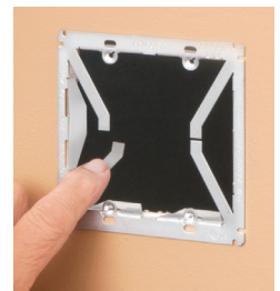
5 Bend all four corner supports into hole and around drywall to set bracket securely in opening.
