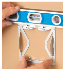
1 Bracket is template for the opening. Place bracket facedown on surface. Level.
