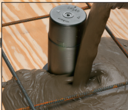
Nail or screw sleeve to form.
