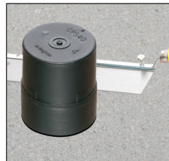
After concrete sets. Cut sleeve off flush with surface.
