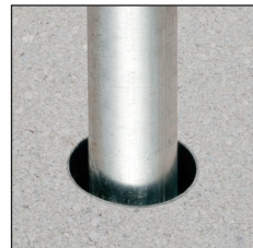
Insert conduit into sleeve.
